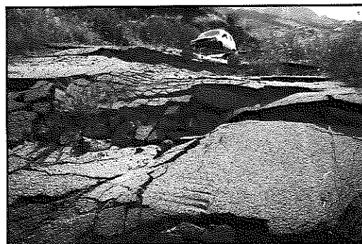
Damage after an earthquake
